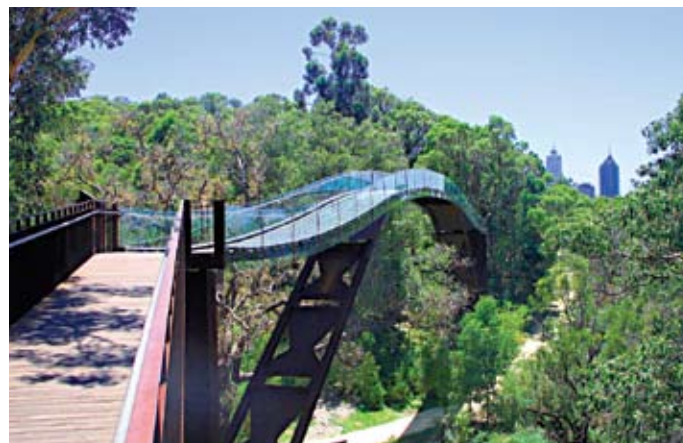
Stezka Lotterywest Federation Walkway v Kings Park
