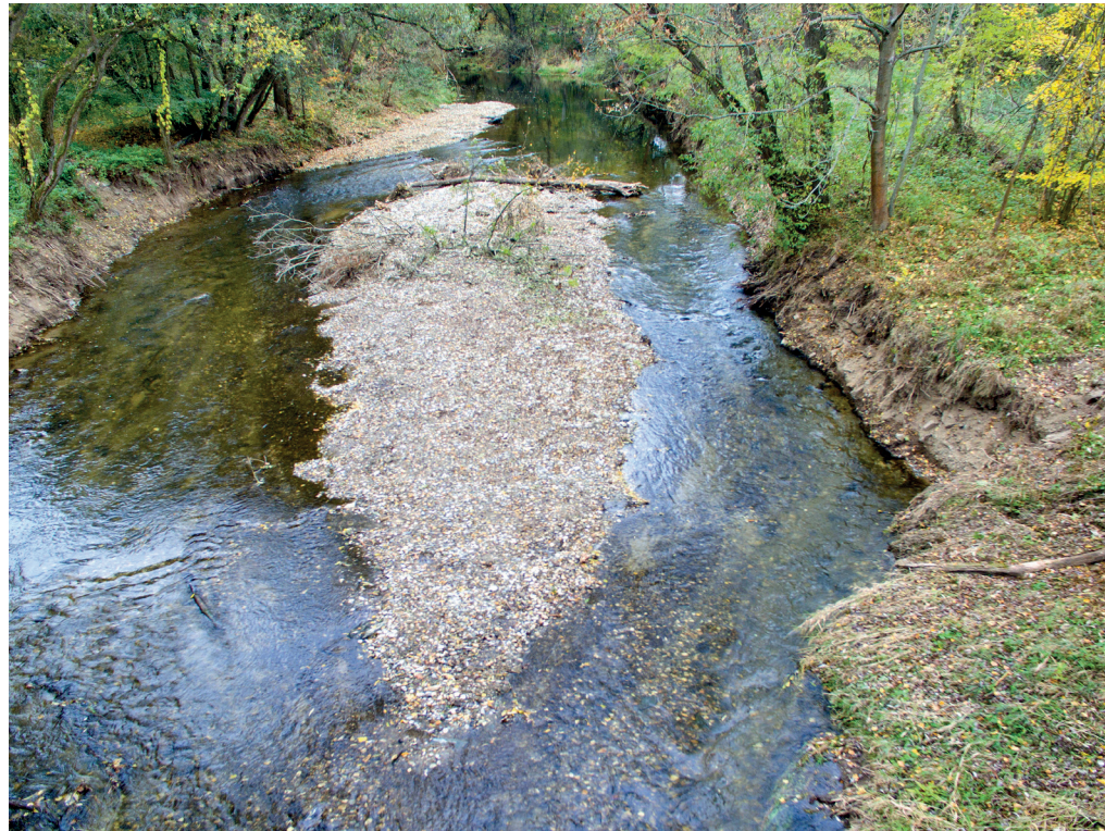
Figure 4: Promoting the restoration of the Morava River near the town of Štěpánov by the removal of historical bank fortification; new elements to divide the channel morphologically and hydraulically were produced from material from the dismantled fortification. © Jan Koutný
