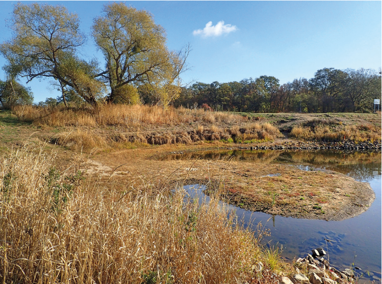
Using historically created groynes (‘Buhnen’) to improve navigation, banks on the German middle Elbe were corrected to their present form, here covered with willows and oaks, with a sand bottom and pools. Photo Petr Bauer
