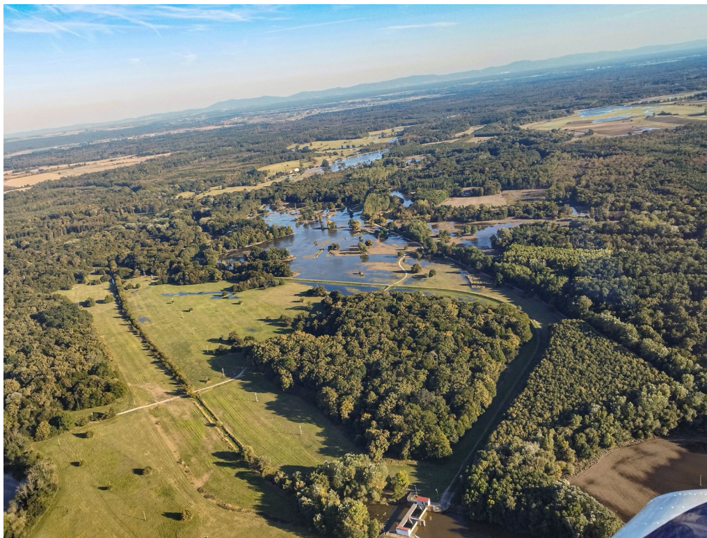
Figure 4. Pohansko weir, 22 September 2024, the day the flood peak subsided. © Adam Koukal During the September 2024 floods, Pohansko weir (at the lower edge of the image) was not used to inundate the alluvial forest. Floodwaters are largely confined outside the polder, and the embankment paradoxically prevents Dyje/Thaya River floodwaters from spreading into the polder.
