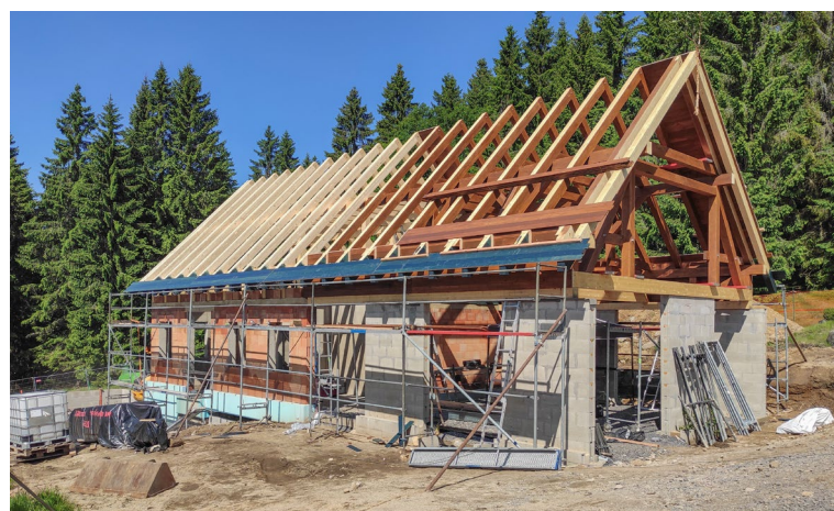
Figure 8. Building the Jizerské hory/Jizera Mountains Protected Landscape Area Information Centre – Mariánskohorské Boudy/Maria Hills Cabins (northern Bohemia) is co-financed by the National Recovery Plan and will open to the public in the spring of 2026. © Daniel Kopecký
